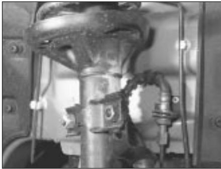
2.4 Disconnect the brake hose from the front suspension strut
